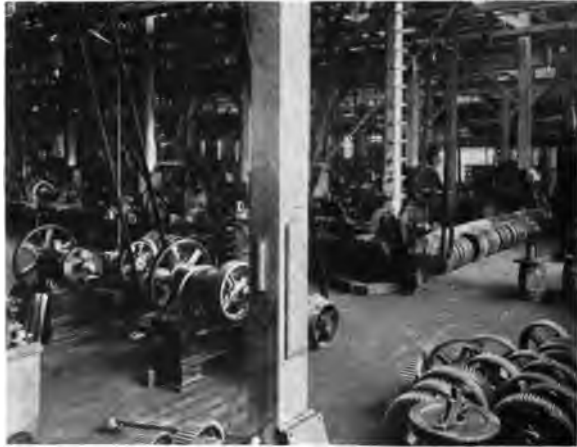
View in Gear Cutting Department
